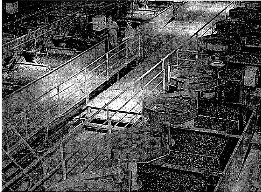
Installation of Knelson Concentrators at Bimak AD, Bulgaria
